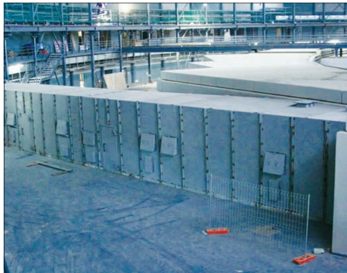
ALBA's main building is built on a hard floor floating on a bed of gravel.
